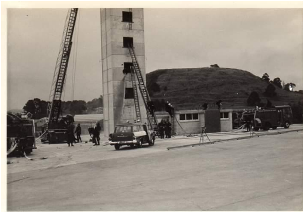
Training Centre Tower and Smoke Chamber
